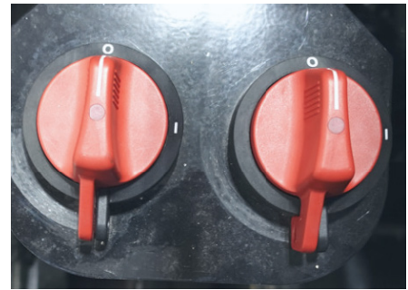
Figure 10. Switches in off position
