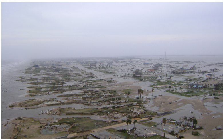
Above left: Houses on North Galveston Bay were inundated. Damage was widespread. Left: Air crews surveying Goat Island and Crystal Beach shortly after Ike passed found standing water and few structures where once there had been hundreds. (Photos taken by DPS Aircraft Flight Crew 108.)
