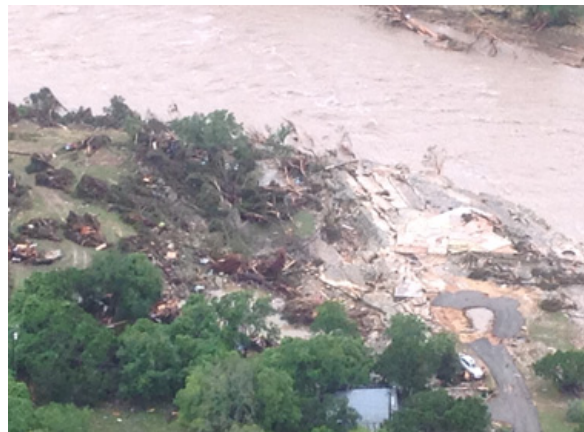
Remains of a home on the Blanco River near Wimberley.
