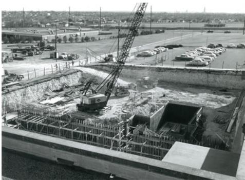
Construction of the [SOC](#) began in 1962, and, due to tensions of the Cold War, the entire structure was contained within a shock absorbing concrete box and buried deep in the limestone and caliche of north central Austin. Protected by large, steel blast doors, the structure was designed to withstand the nearby hit of a 20-megaton nuclear blast.
